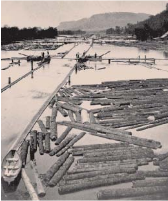
To create log rafts, workers in Beef Slough near Alma, Wis. construct chutes. Log rafts could be more easily pushed downriver to sawmills.
